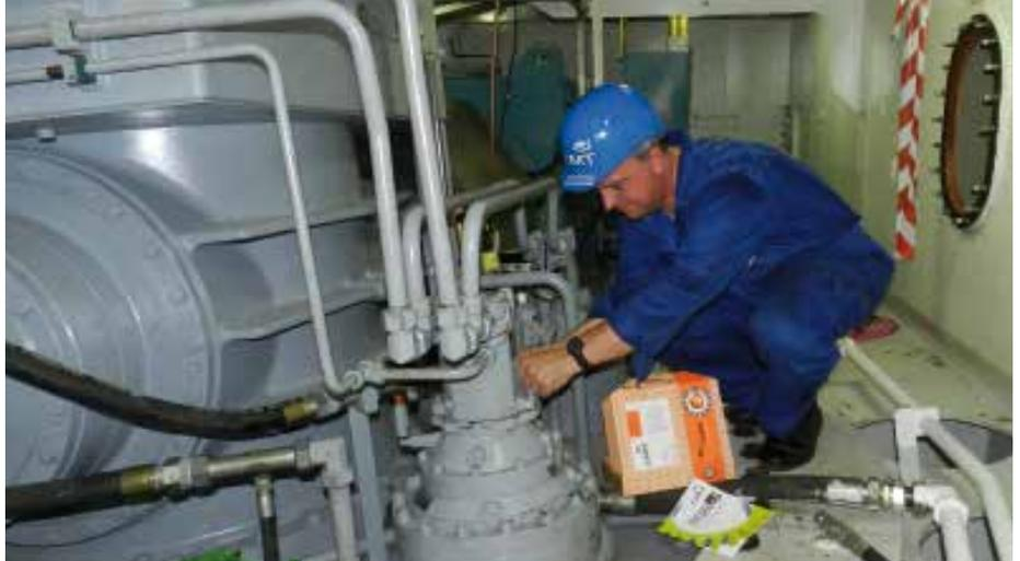
*Removal of a representative oil specimen from the engine of a marine engine.*
