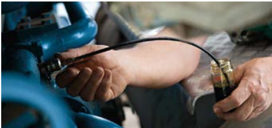
Regular sampling and checking of the gas engine oil, as shown in the photo, is not sufficient. Tectrol generally advises analysing the coolant after a maximum of 2,000 operating hours.
